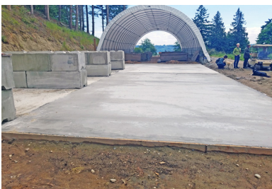
After: Cost-shared BMPs include installing a livestock waste storage facility and heavy use area protection.
