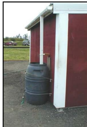
The remaining winter paddock area was planted to pasture. Roof runoff water is directed into a sealed rain barrel, where it is then used to fill a small stock tank. Excess roof runoff water is piped into the newly planted pasture.
