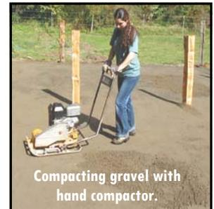
Compacting gravel with hand compactor.
