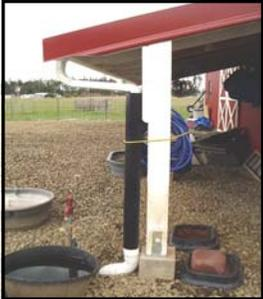
Downspout carries roof water via pipe to drywell.
