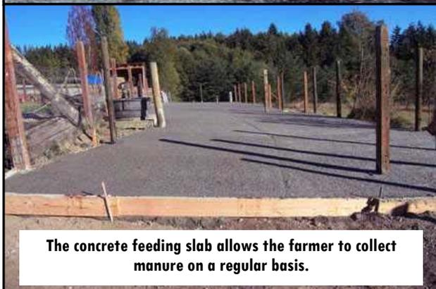
**The concrete feeding slab allows the farmer to collect manure on a regular basis.**
