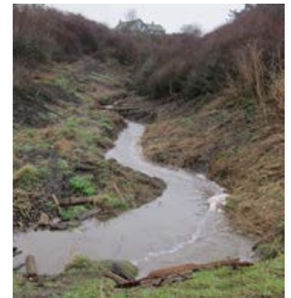
Stormwater drainage discharges into Puget Sound at Ebey's Landing.
