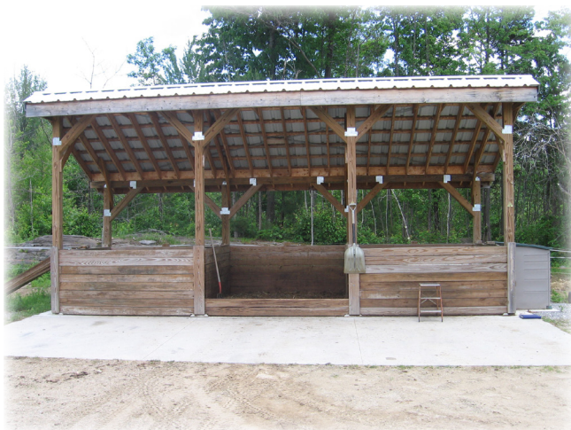
Roofed composting system on concrete pad.
