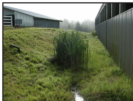
A small swale planted with wetland plants, where roof runoff is outleted to facilitate filtering and infiltration.
